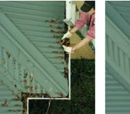
After installation, regularly check for the build-up of debris. If cleaning is needed, say after four months, then that would be your regular maintenance period. Talk to your local handyman if you are unable to check or clean the guttering yourself.
